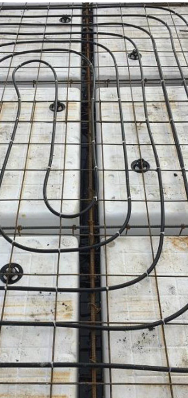
Figure 1: Pre-piping for in-slab underfloor heating
